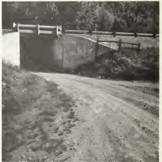
South entrance, looking North
